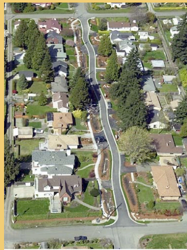
SEA Streets - After Construction 2nd Ave NW - NW 117th St to NW 120th St
