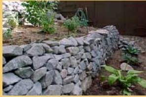
Rock retaining wall
