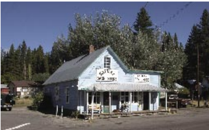
This RCC market and post office are located on a major rural intersection.
