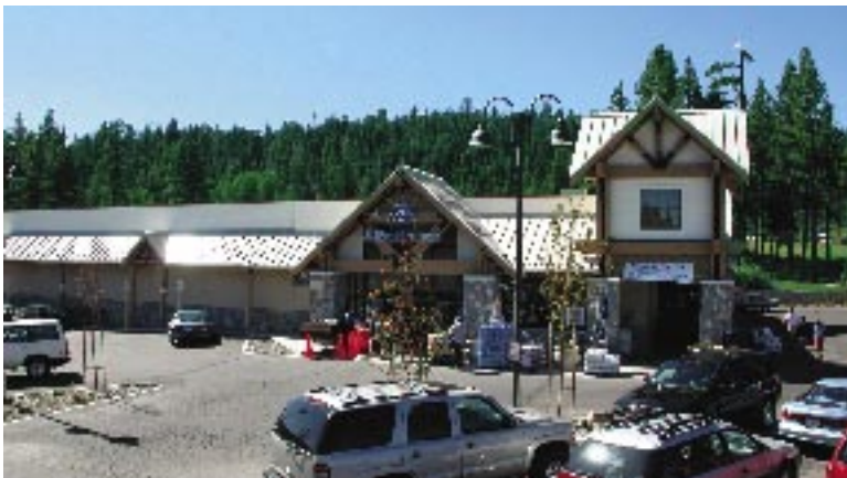
A remodel of an existing SD better reflects the alpine community character of Tahoe City.
