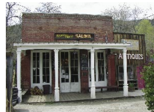
Genoa showcases Sierra architectural standards in the oldest bar in Nevada.
